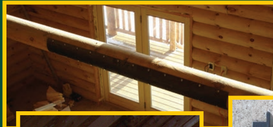
Coped Tie Beam Strap
