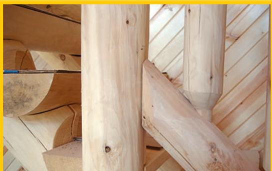
← Bevel Cut A bevel cut is made on both sides of the top and bottom rail before attaching to the posts.
