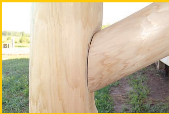
Cope Support Post Shave the support post down with a planer or sander. Attach rails.
