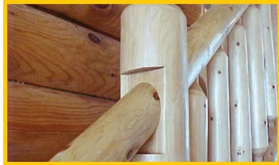
Router then chissel out a small area on the support post where the top and bottom rails will meet. Use a belt or finish sander to sand the area flat.
