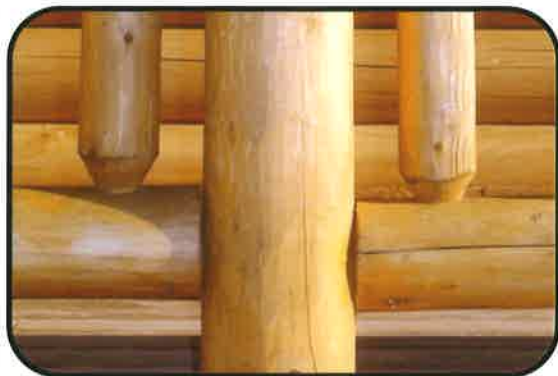
Square Cut This is the easiest method for attaching square cut railing. Top and bottom rails butt up directly to the post.
