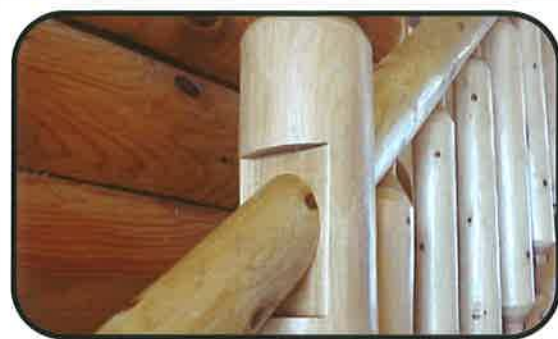
Router then chisel out a small area on the support post where the top and bottom rails will meet. Use a belt or finish sander to sand the area flat.
