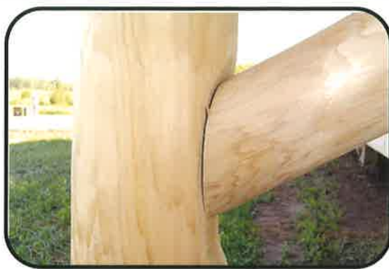
Cope Support Post Shave the support post down with a planer or sander. Attach rails.
