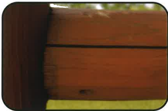
Cope Top and Bottom Rail Use a coping saw, sawzall, or jigsaw to cope the top and bottom rails. Attach to support posts.
