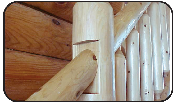
Router then chissel out a small area on the support post where the top and bottom rails will meet. Use a belt or finish sander to sand the area flat.
